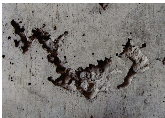
Fig. 2. Macro-sized voids on the concrete surface.
